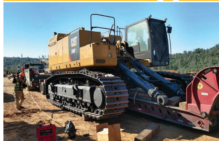
Peterson onsite service during Oroville Dam spillway project
