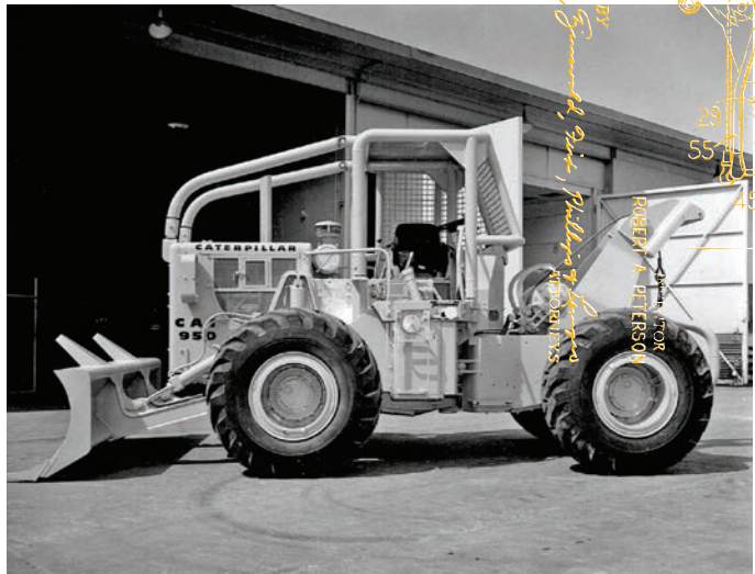
Buster's experimental 905 wheel skidder made from a 950 wheel loader in 1968
