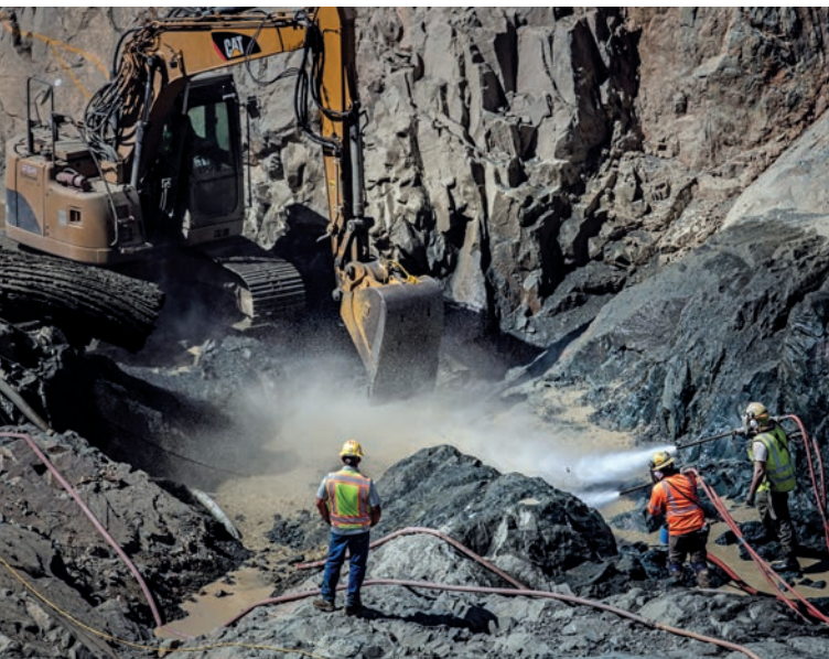
Left to right: Meticulous cleaning of bedrock to insure a clean bond between concrete and rock in September 2018; Breaking up the first season's temporary walls of roller-compacted concrete (RCC) in May 2018
