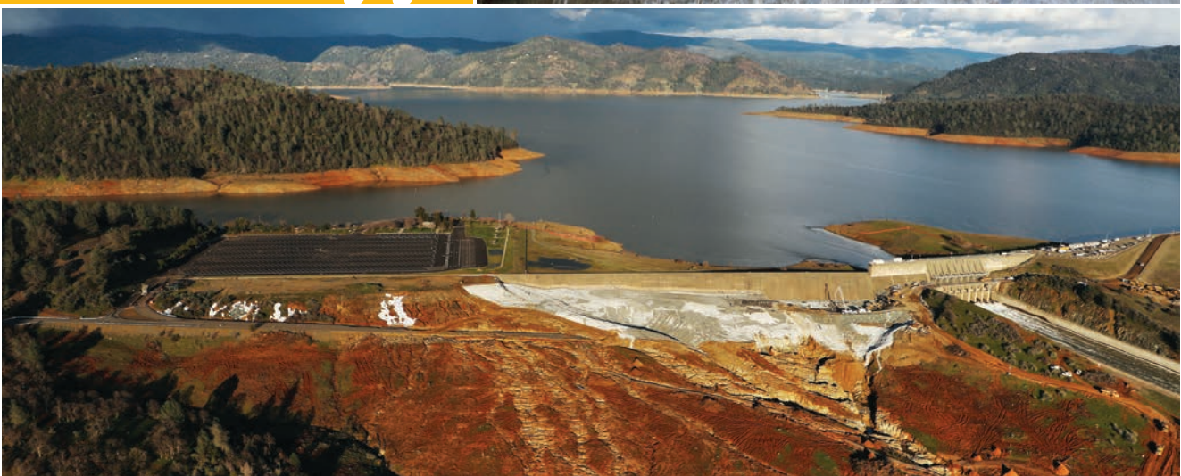
The aftermath of the Oroville spillway break in the spring of 2017
