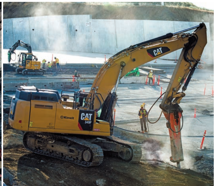
Left to right: Meticulous cleaning of bedrock to insure a clean bond between concrete and rock in September 2018; Breaking up the first season's temporary walls of roller-compacted concrete (RCC) in May 2018
