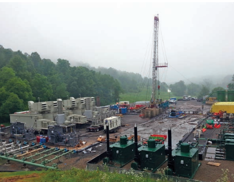
Fracking site with four Solar Turbines
