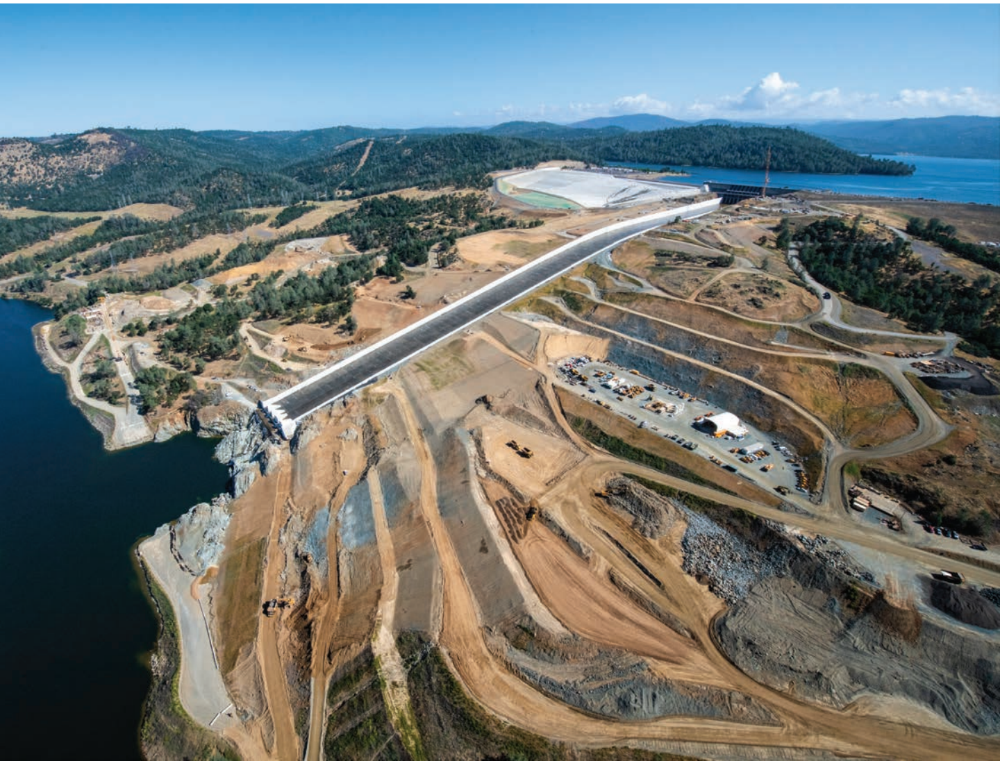
Kiewit's Oroville Dam spillway project near completion in June 2019
