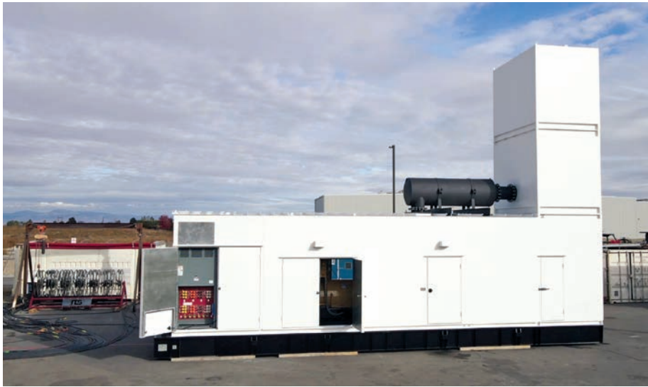
Left to right: Typical backup generator system housed inside special enclosure; Close up of Cat 3516 generator inside enclosure with (L-R) Bob Tanzer & Gene Hamilton
