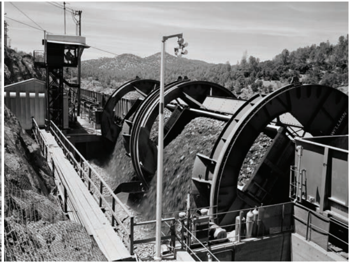
Left to right: Two of Buster's original Quad D9s (No. 107 & 109) were used on the Oroville Dam project in 1964-65; Oman used a railroad system with automated railcar tippers to transport materials instead of a traditional fleet of scrapers and haul trucks.
