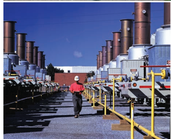
Top to bottom: Gene Hamilton with Bruce Baxter of Toromont at Markham site in 2003; Markham mobile turbine power plant in Toronto.
