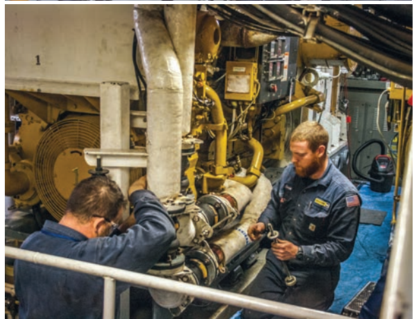
Peterson marine techs work in tight quarters
