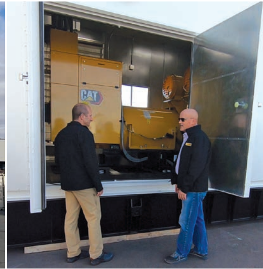
Left to right: Typical backup generator system housed inside special enclosure; Close up of Cat 3516 generator inside enclosure with (L-R) Bob Tanzer & Gene Hamilton
