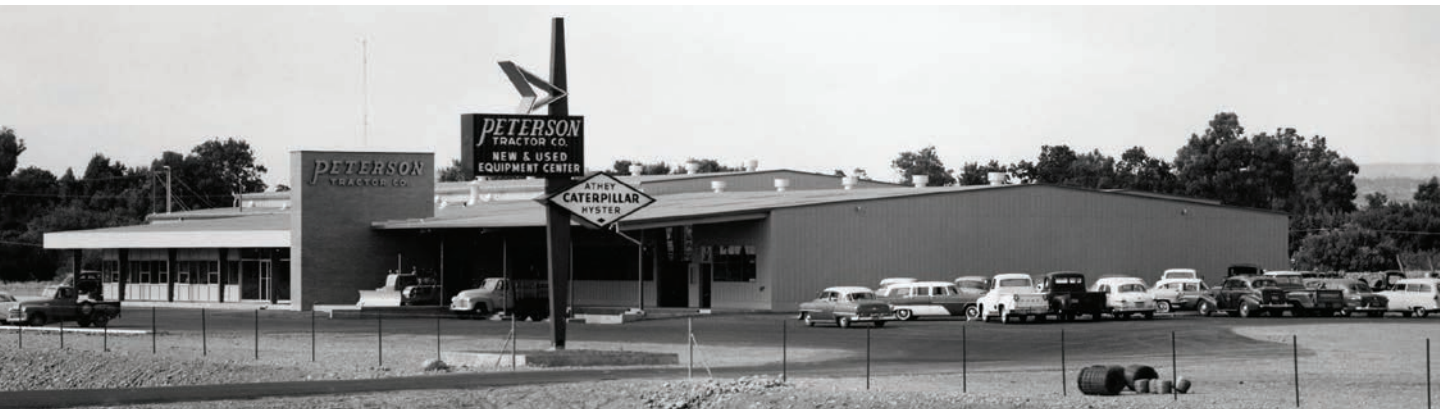
Peterson moved into its new Chico facility on July 1, 1958 to serve the Oroville Dam project and local customers.
