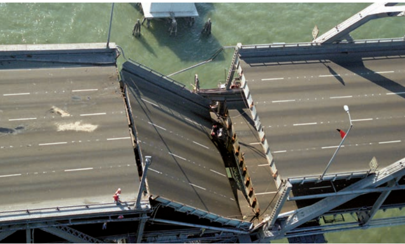
Left to right: Car caught in a collapsed section of the SF-Oakland Bay Bridge in 1989; Loma Prieta earthquake 'pancaked' the Cypress Structure on I-880 in Oakland, California in 1989
