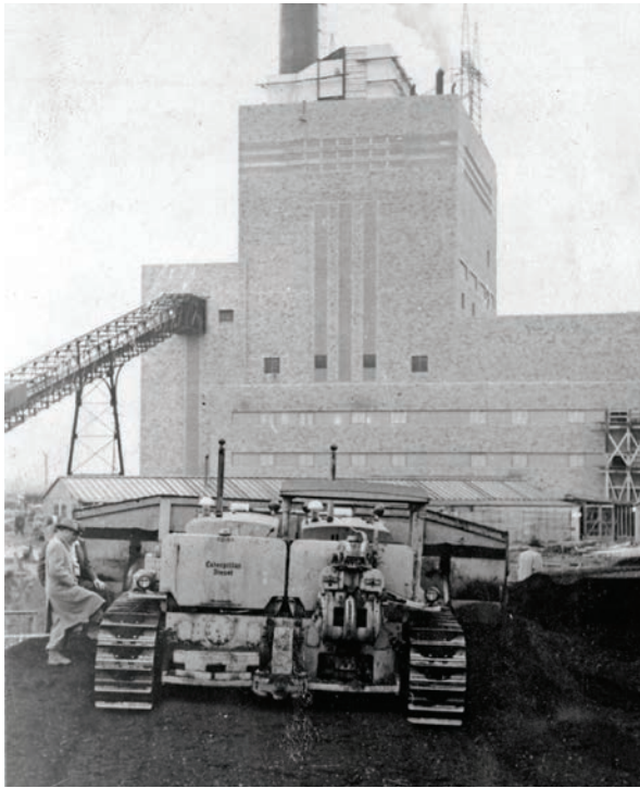
Coal Twin keeps stacks fed at Tanners Creek Power Plant circa 1950s
