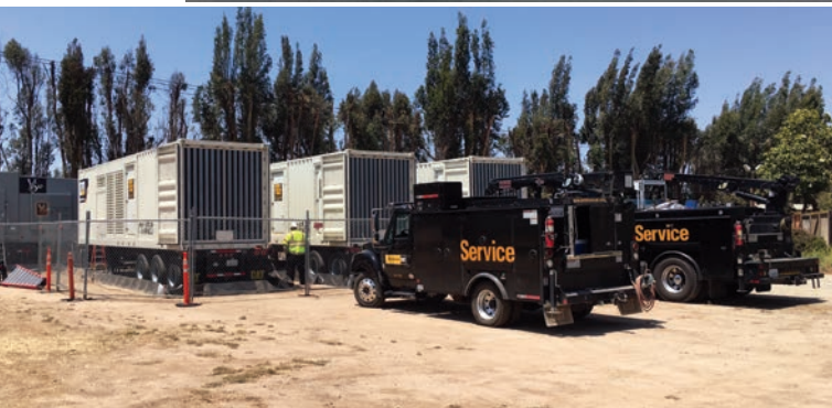
Rental generator lineup & power modules onsite
