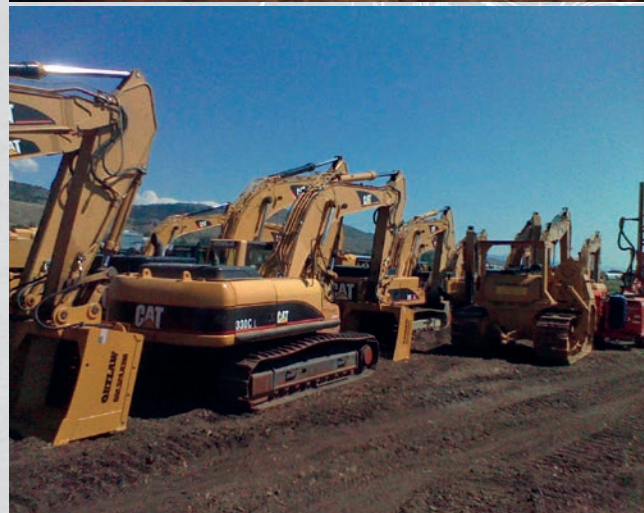
Peterson had 300 Cat rental machines on the job, between Spreads 6 & 7
