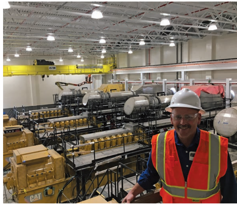
Gene Hamilton at a cogeneration site in San Jose, California in 2019
