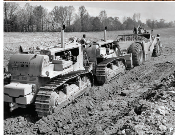
Top to bottom: Article about I-64 job in Virginia; Oman Quads used on I-64 contract in Covington, VA in June 1964; S.J. Groves using one of Buster's original Quad D9s
