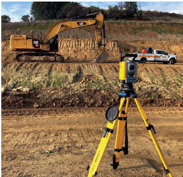
Machine control technology used on the Oroville Dam spillway project
