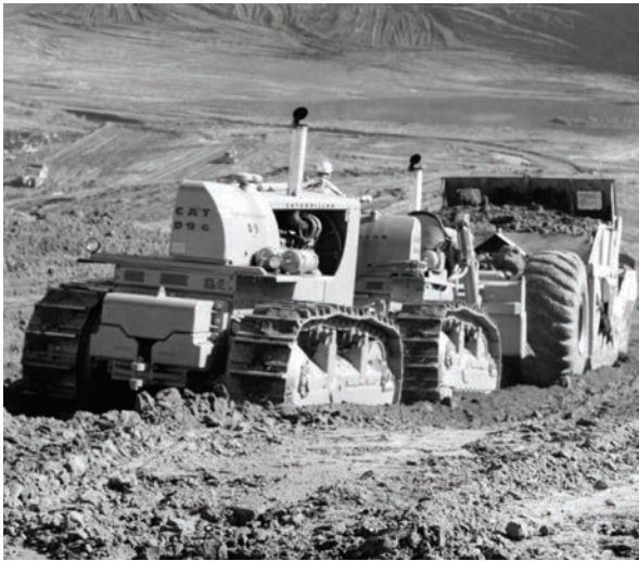
Left to right: Two of Buster's original Quad D9s (No. 107 & 109) were used on the Oroville Dam project in 1964-65; Oman used a railroad system with automated railcar tippers to transport materials instead of a traditional fleet of scrapers and haul trucks.
