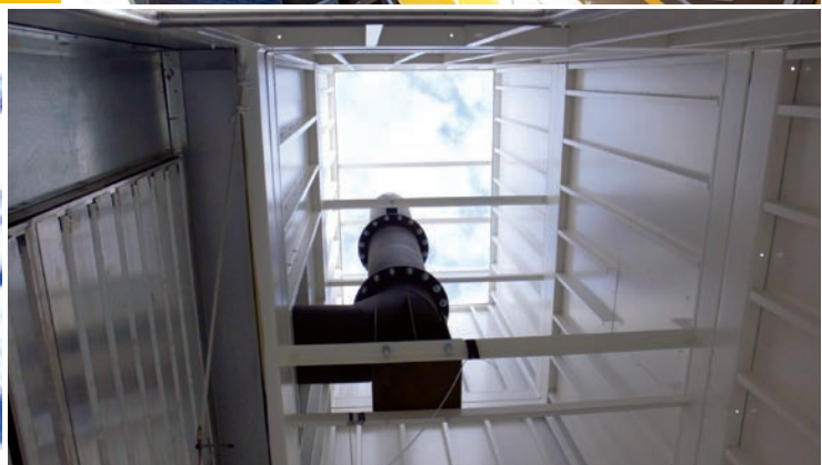
Top, clockwise: Packager Johnson Thermal Systems building enclosures; Cat generator inside enclosure; Plenum (tower) of exhaust system external & internal view
