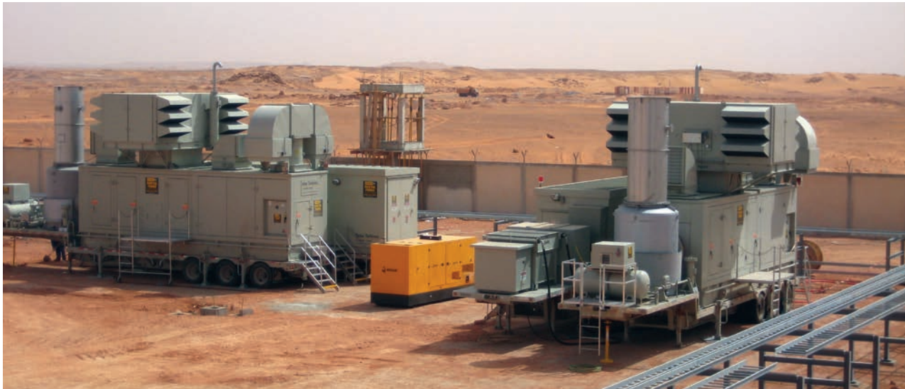
Turbine installation in Algeria
