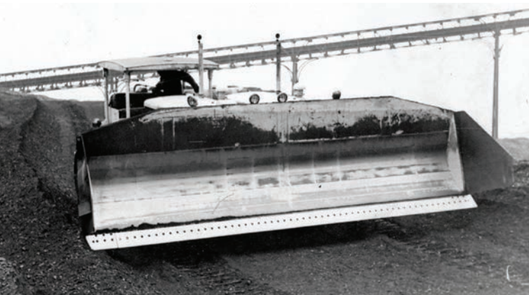
The Coal Twin at Tanners Creek Power Plant circa 1952
