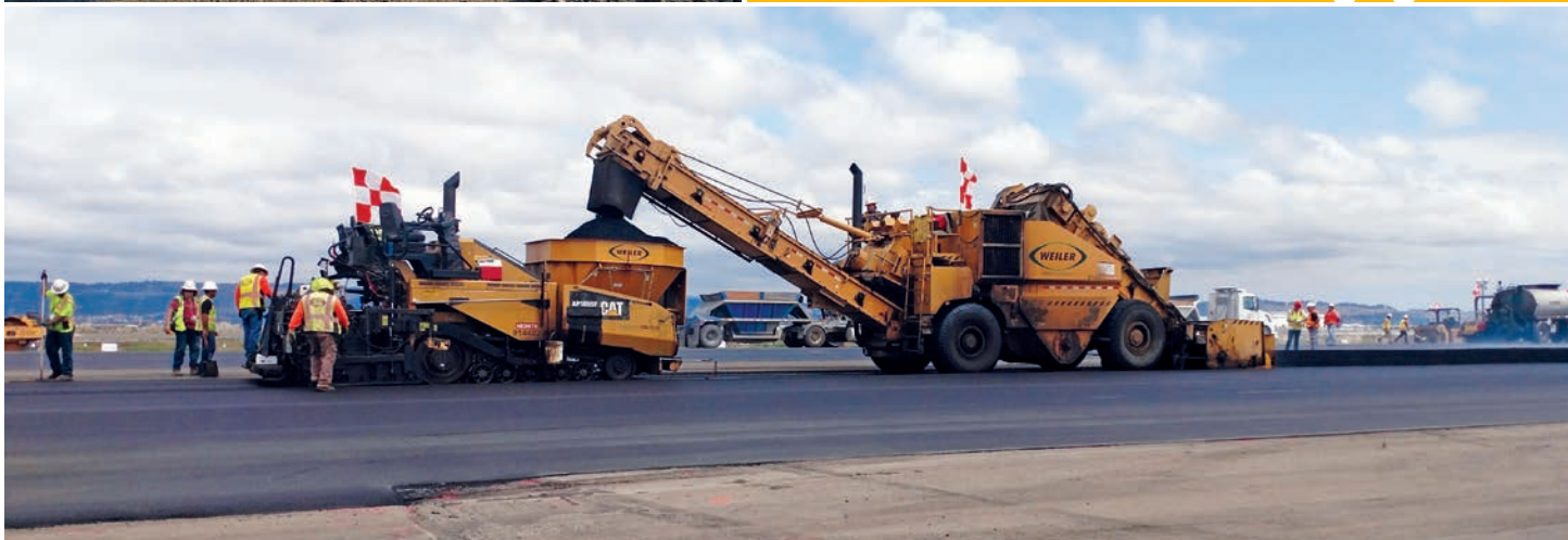
Top to bottom: Rich Poppoff/L. during paver training; DeSilva’s Cat AP1055F paver; DeSilva’s Cat paver with Weiler MTV machine
