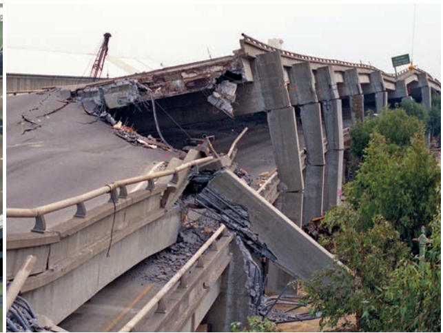
Left to right: Car caught in a collapsed section of the SF-Oakland Bay Bridge in 1989; Loma Prieta earthquake 'pancaked' the Cypress Structure on I-880 in Oakland, California in 1989
