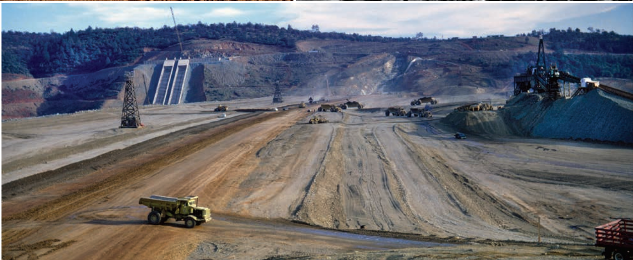
Original construction of Oroville Dam in the 1960s. Buster-built Quad D9 pictured at top. (Center) Oman used a giant wheel excavator to harvest the old mine tailings for fill material on the dam.
