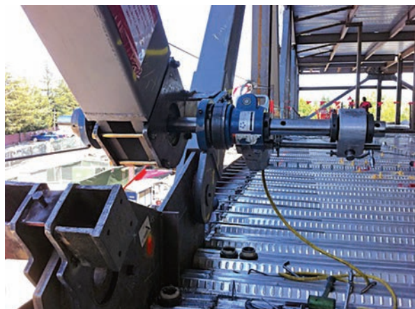
Portable boring bar in place for re-aligning miss-matched holes in crossbeams
