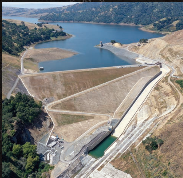
Calaveras Dam Rebuild during (top) and after (above)
