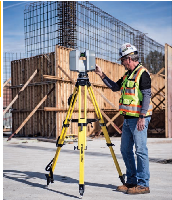
BuildingPoint’s Trimble 3D laser scanner on the job
